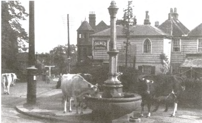
Picture 2.78 Historic cattle trough when it was located in the Stanmore Hill Conservation Area, but which is now located in the Old Church Lane Conservation Area
