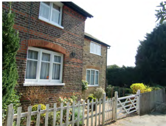
Picture 2.67 Timber casement windows and brick banding detail along Green Lane
