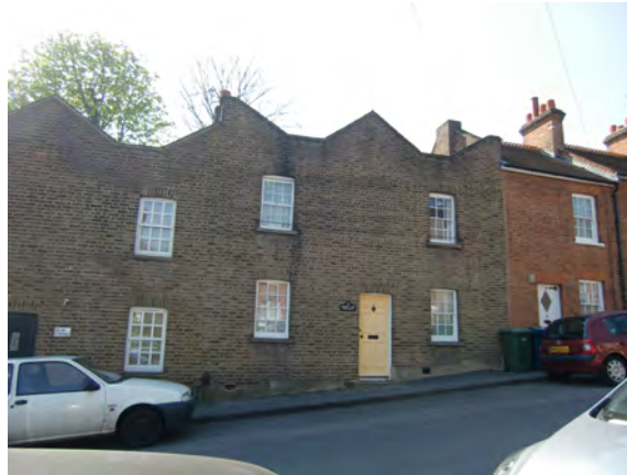
Picture 2.56 Nos. 1-4 Green Lane are unified by their angular parapet wall, also known as a Butterfly Roof
