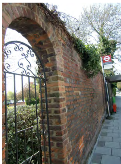
Picture 2.66 Historic brick wall outside Halsbury Court, Stanmore Hill
