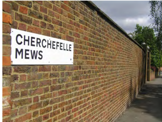
Picture 2.25 Important historic brick wall of Cherchefelle Mews fronting public highway, lower reaches of Green Lane
