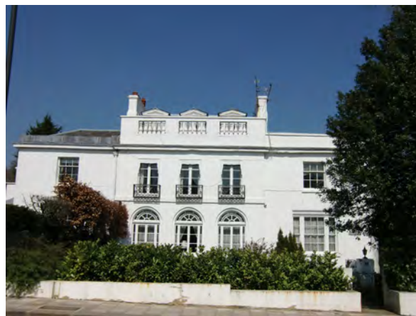
Picture 2.33 Grade II listed Goodengate, Stanmore Hill
