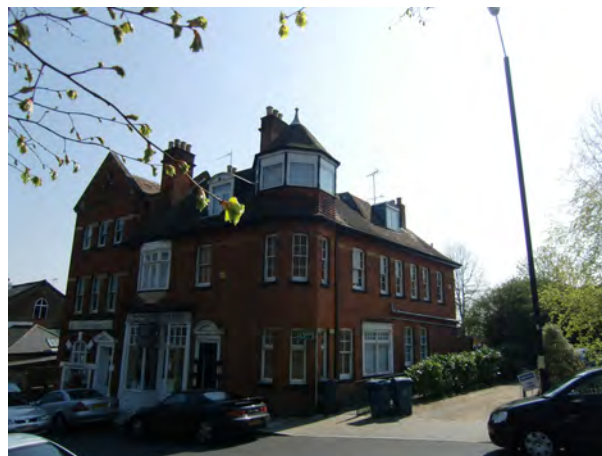
Picture 2.41 Locally listed nos.103 to 107 (odd) Stanmore Hill
